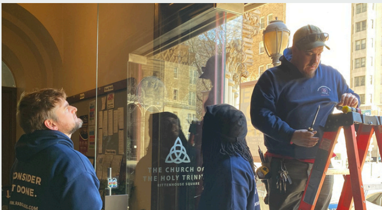
Replacing the glass front doors
