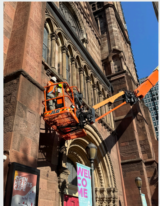
Repairing damage to the roof of the church's bell tower
