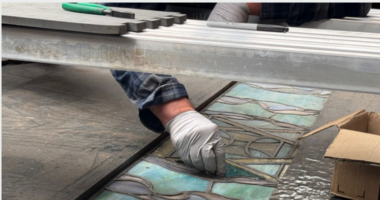
Contractors working on the Tiffany glass in the Sanctuary Dome laylight
